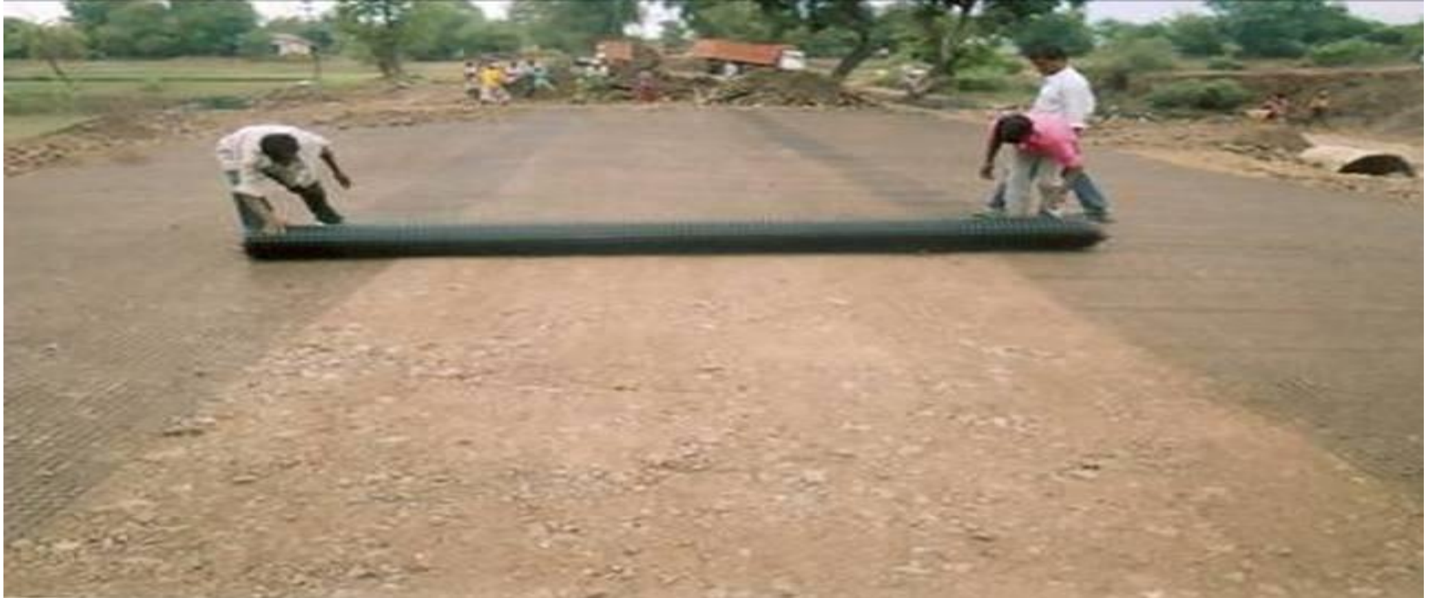
Subgrade Stabilization using Tensar Biaxial Geogrids Talasari - Udhava Major Dist. Road, PWD, Maharashtra
