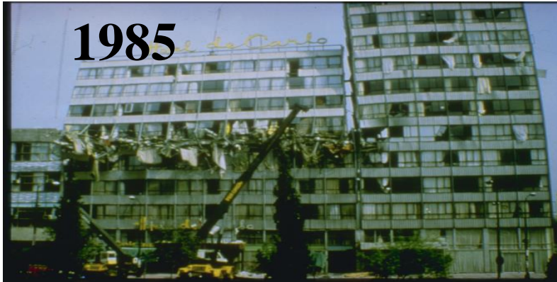
Earthquake Damage in Mexico City, Mexico, September 19, 1985 - resonance
