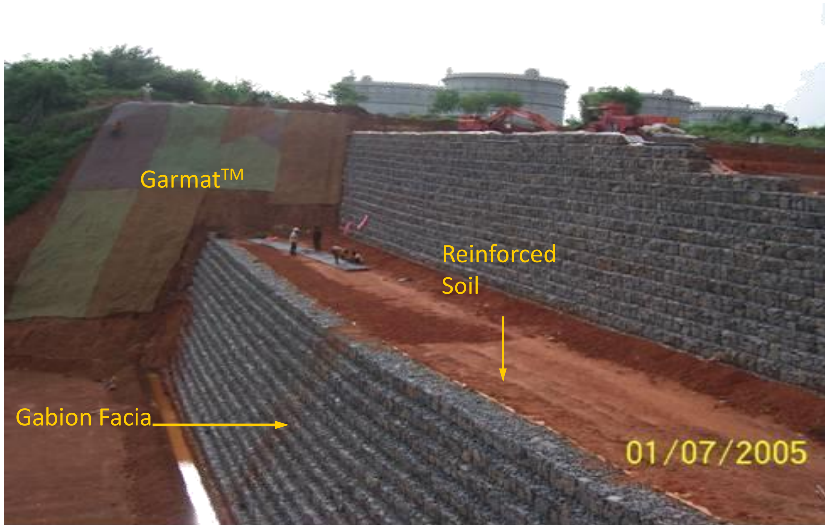
Reinforced Soil System with Gabion Fascia, MRPL, Mangalore
