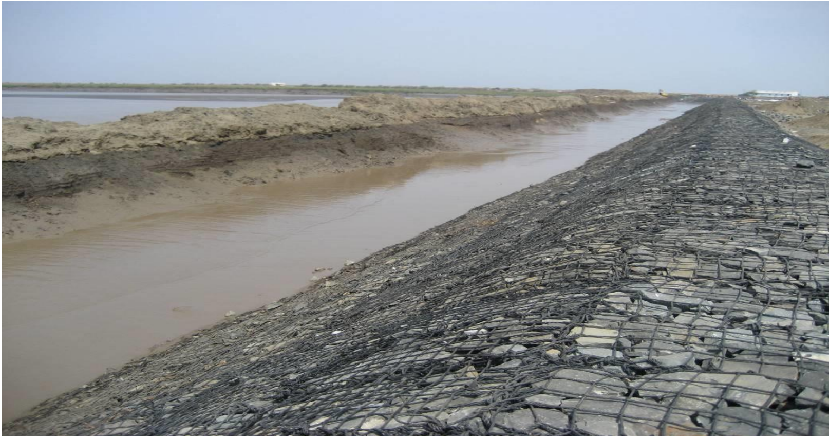
Revetment - Anti Erosion Sea Bund Morbhagwa, Gujarat, India
