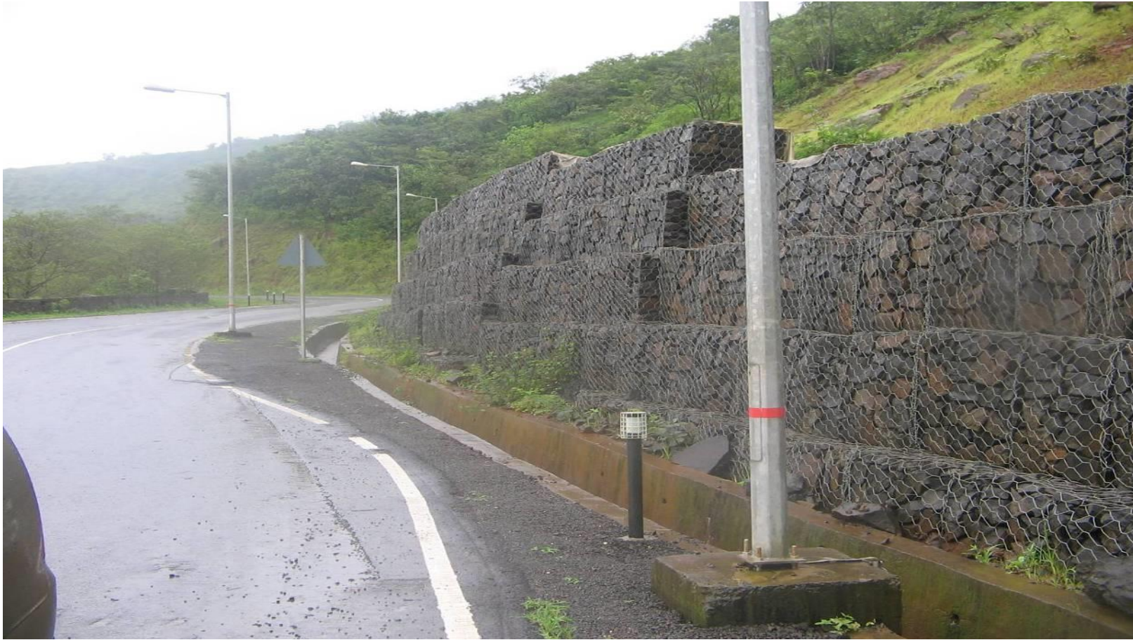
Gabion Retaining Wall – Lavasa
